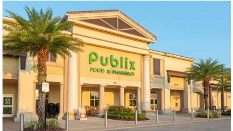
Nocatee Town Center | Jacksonville, FL
