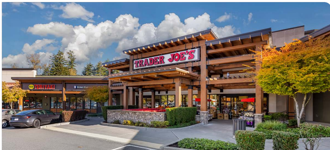
Sammamish Highlands | Seattle, WA
