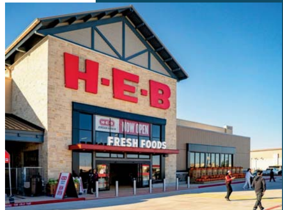
Jordan Ranch Marketplace Houston, TX 2025 Development Completion
