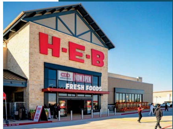
Jordan Ranch Marketplace Houston, TX 2025 Development Completion
